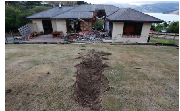
New Zealand Earthquake
